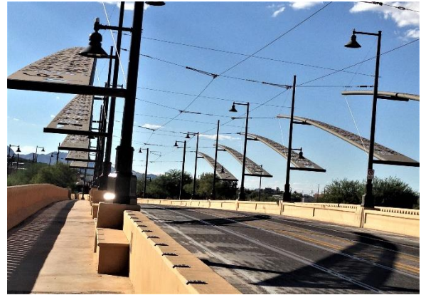
Cushing St/Luis Gutierrez Bridge
